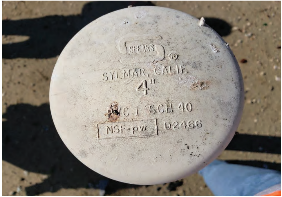
Photograph 11: View of unknown PVC pipe.
