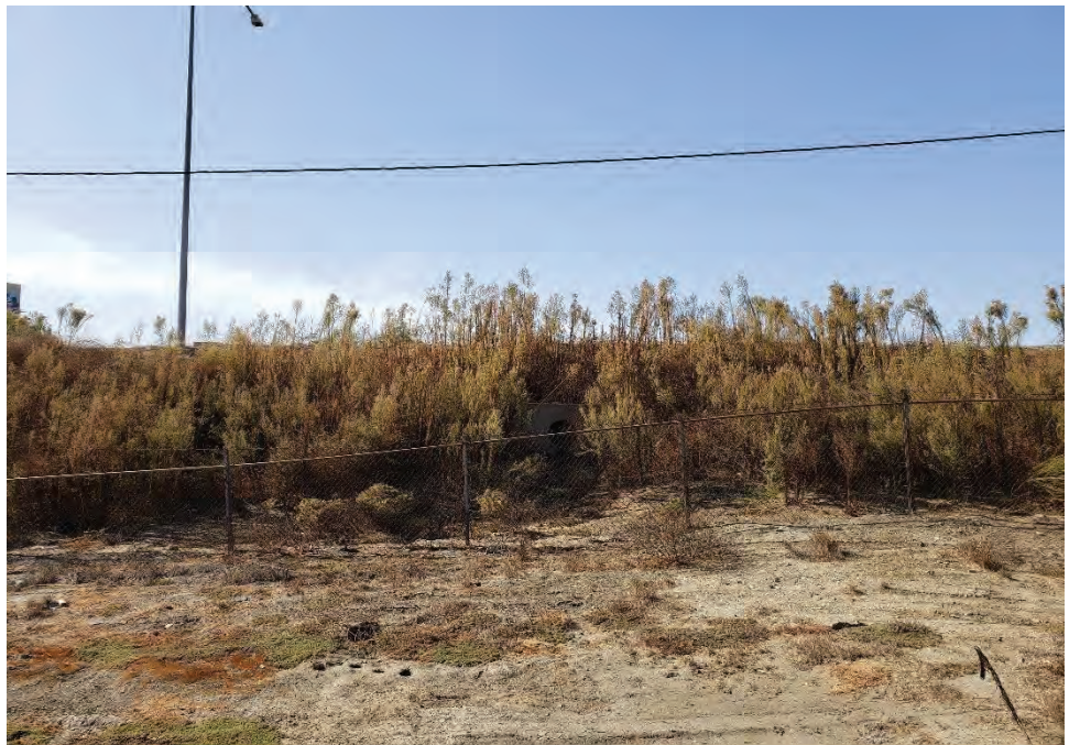
Photograph 8: View of storm drain outlet, under I-405 outside the property.
